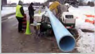
Cold Weather Fusion at -14°C (6°F)
