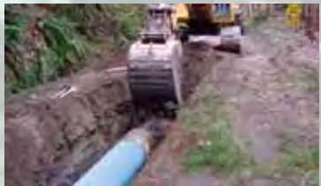
Pipe Pulled In
