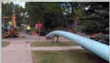
HDD Pipe Insertion
